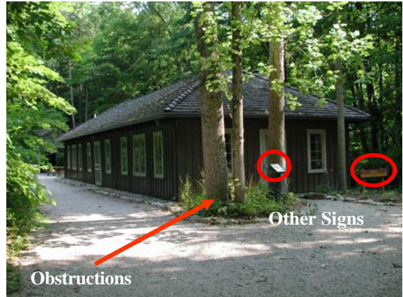
CCC Recreation Hall McCormick's Creek State Park
