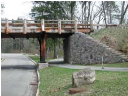
Sign placement takes into consideration road and bike path safety issues.
