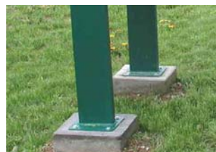
Base plates allow a sign to be more easily removed if necessary.
